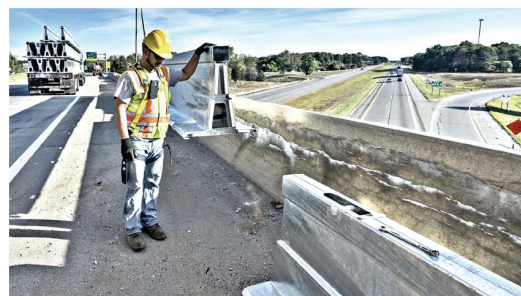
BARRIER SOLUTION FOR BATTLE CREEK BRIDGE Battle Creek, MI | M-66, over I-94
